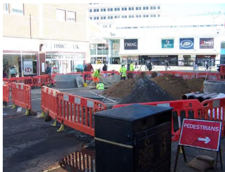
Figure 3: Victoria Plaza Centre
