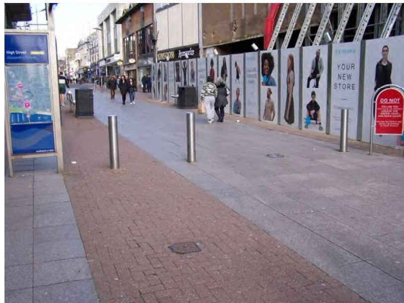
Figure 30: Route 17 impact point. Retractable bollard down allowing vehicular access.
