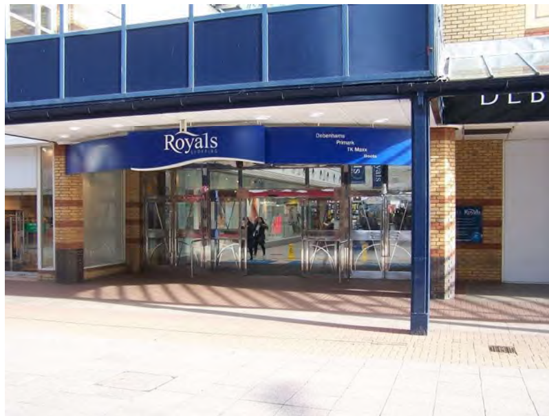
Figure 19: Royal Shopping Exit into the High Street
