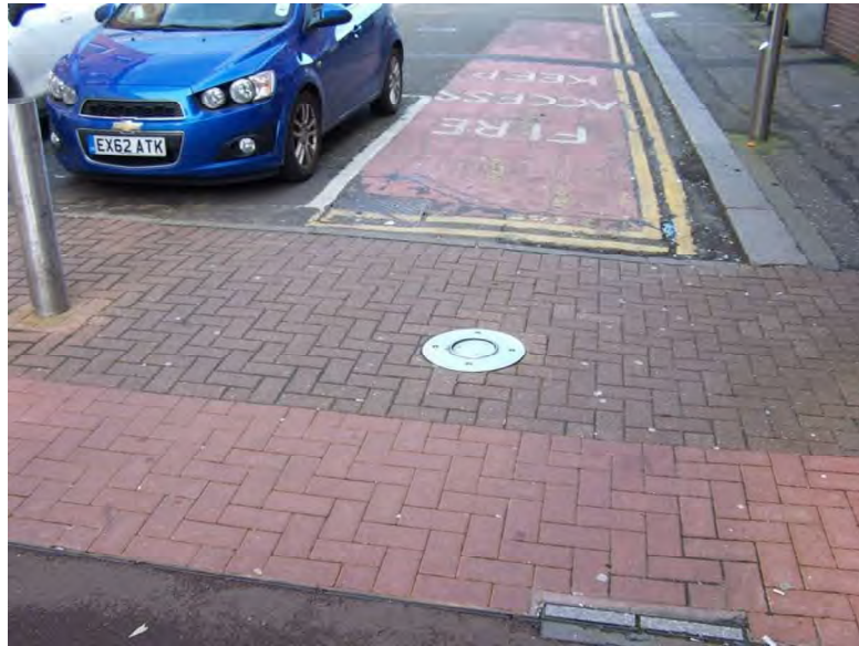
Figure 9: Route 7 impact point retractable bollard
