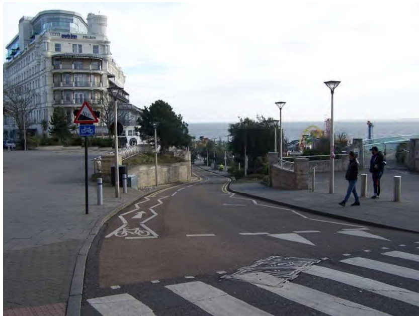
Figure 21: View along Route 12 – Pier Hill – from the impact point
